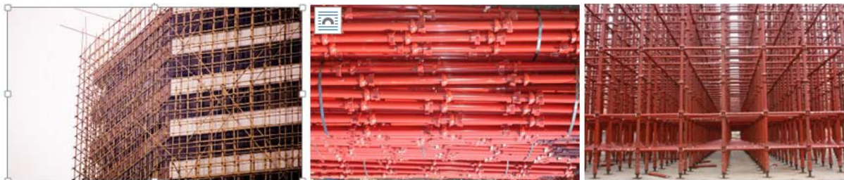
External System scaffolds System scaffolds Birdcage internal scaffolds
