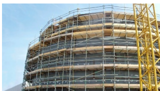
External boiler scaffolds Pre-engineered systems for large or complex projects
